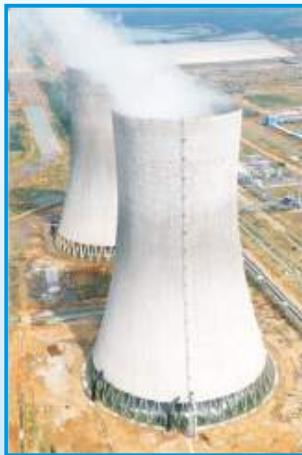
RCC Natural Draft Cooling Tower
