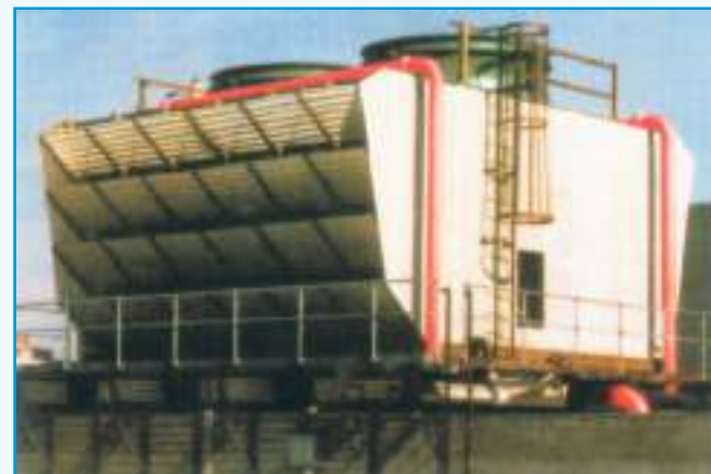
Cross Flow Cooling Tower In Timber Construction
