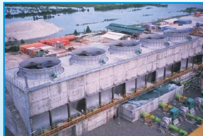
Counter Flow Cooling Tower In RCC Construction
